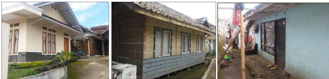
(1) Confined Masonry Building, (2) Non-Masonry Building, and (3) Unreinforced Masonry Building
